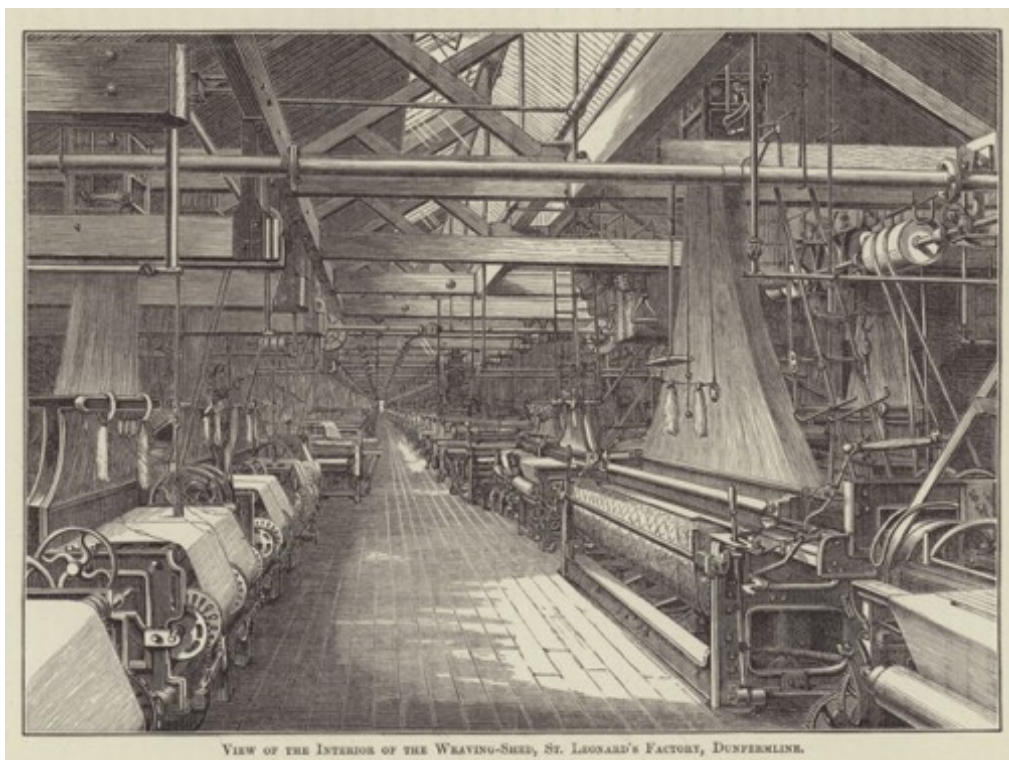
VIEW OF THE INTERIOR OF THE WEAVING-SHED, ST. LEONARD'S FACTORY, DUNFERMLINE.
